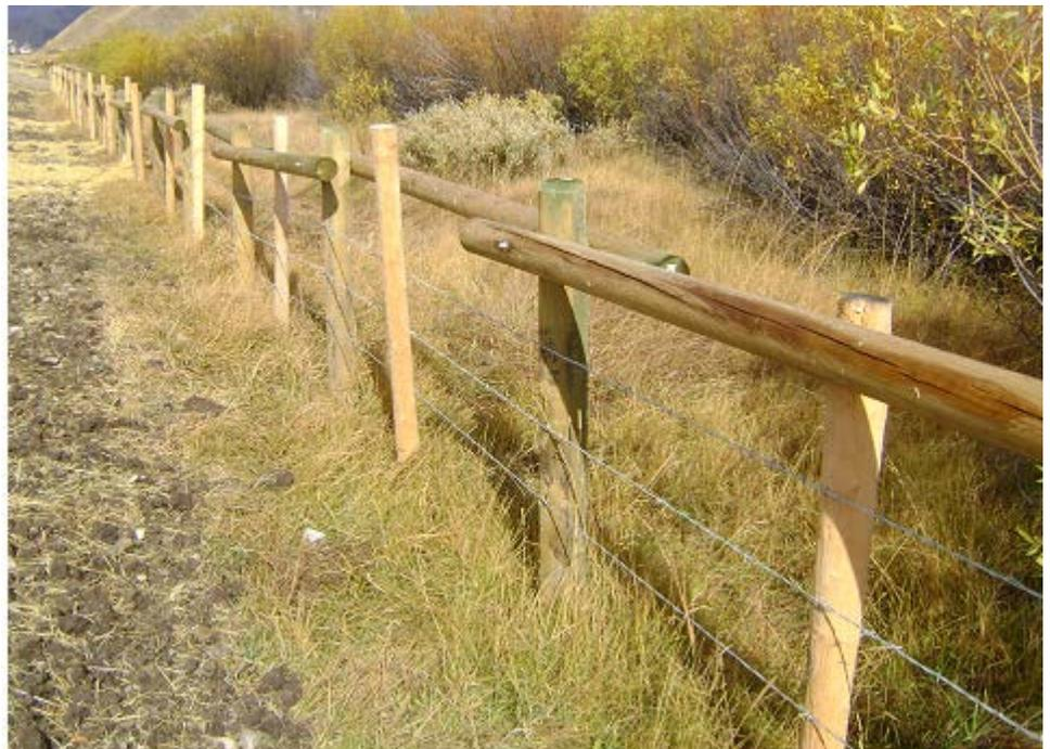
*Roundwood fence alongside the newly constructed Wyoming highway. Treated fence posts are holding up wire and alternating top rails. Roundwood stays are placed between each post to keep the wire up in deep, heavy snows. Photo by Craig Rawlings*
